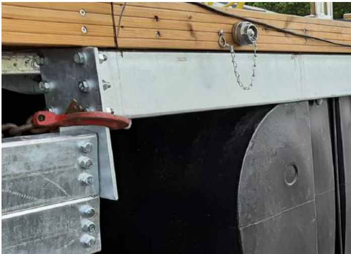
WASTE PUMP CONNECTION
